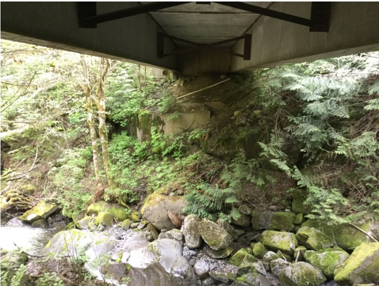
Right Bank Abutment when facing downstream
