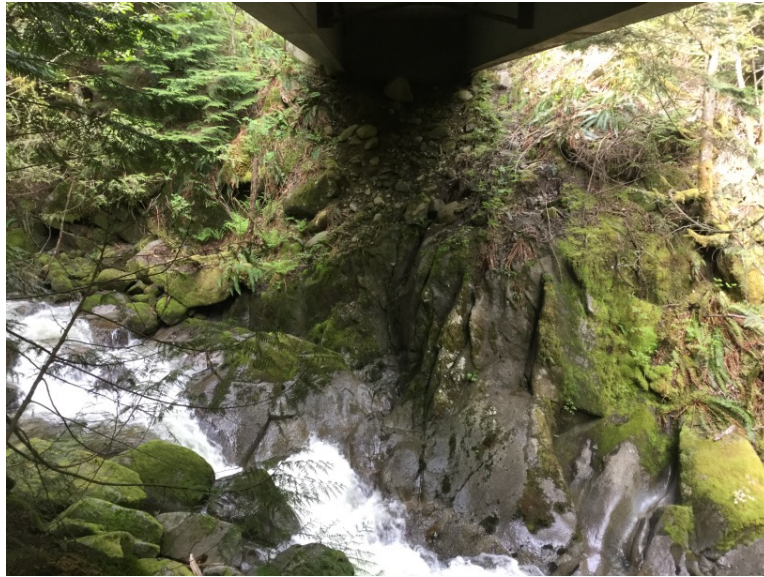
Left Bank Abutment when facing downstream
