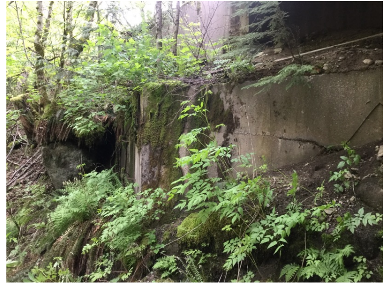
CIP fill retention system at downstream right bank
